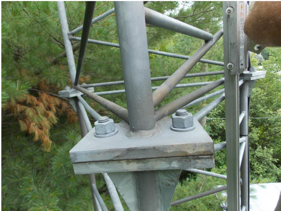
37 Splice Level Two
