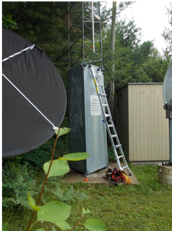
28 Tower Base Azimuth Two
