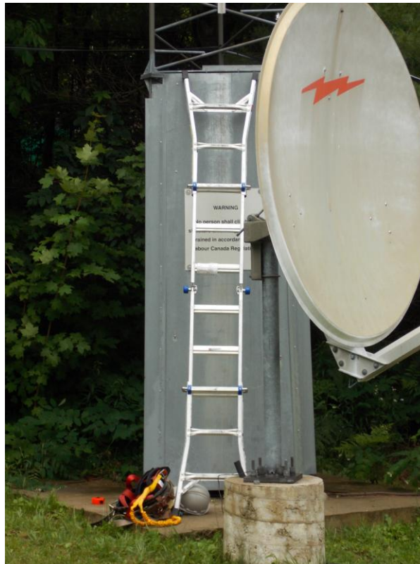
17 Tower Base Face One
