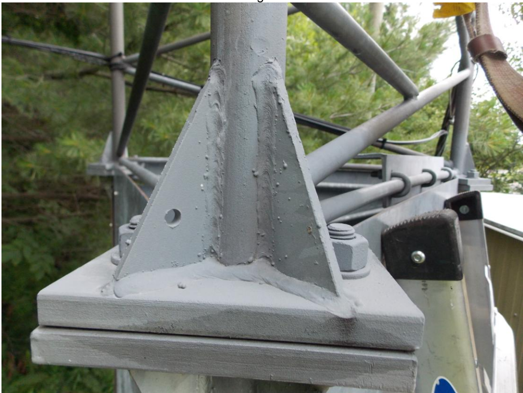
36 Splice Level One
