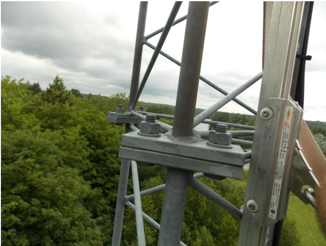
41 Splice Level Six
