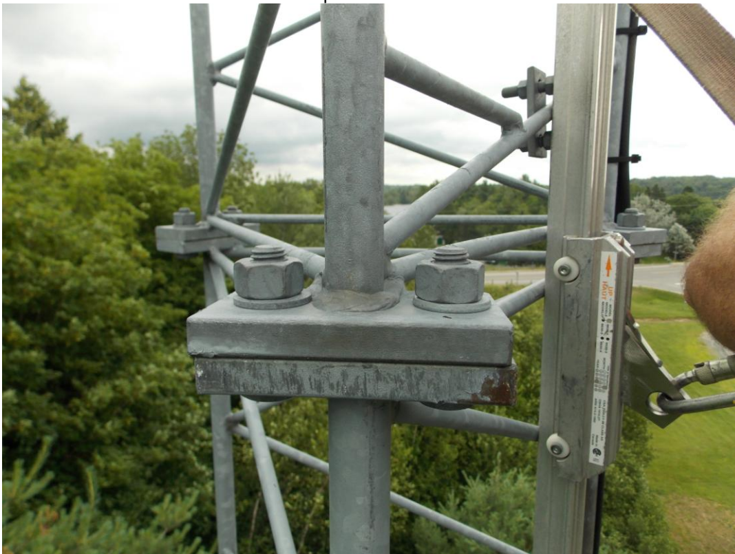
40 Splice Level Five
