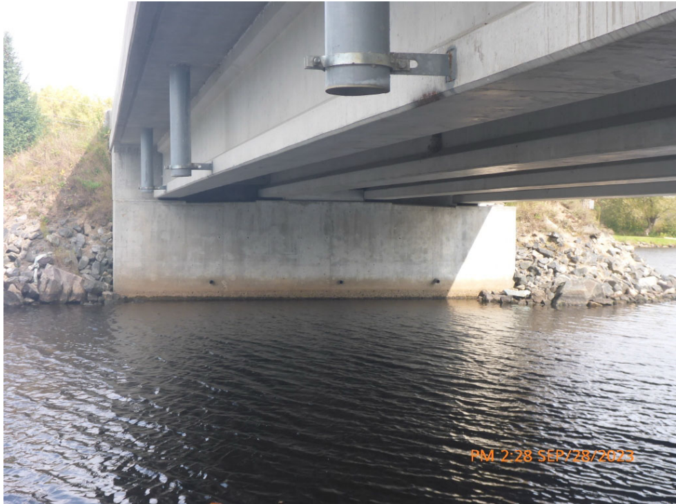
Comments: TYPICAL NORTH ABUTMENT Path: P:\McKellar\2023\P1080257.jpg
