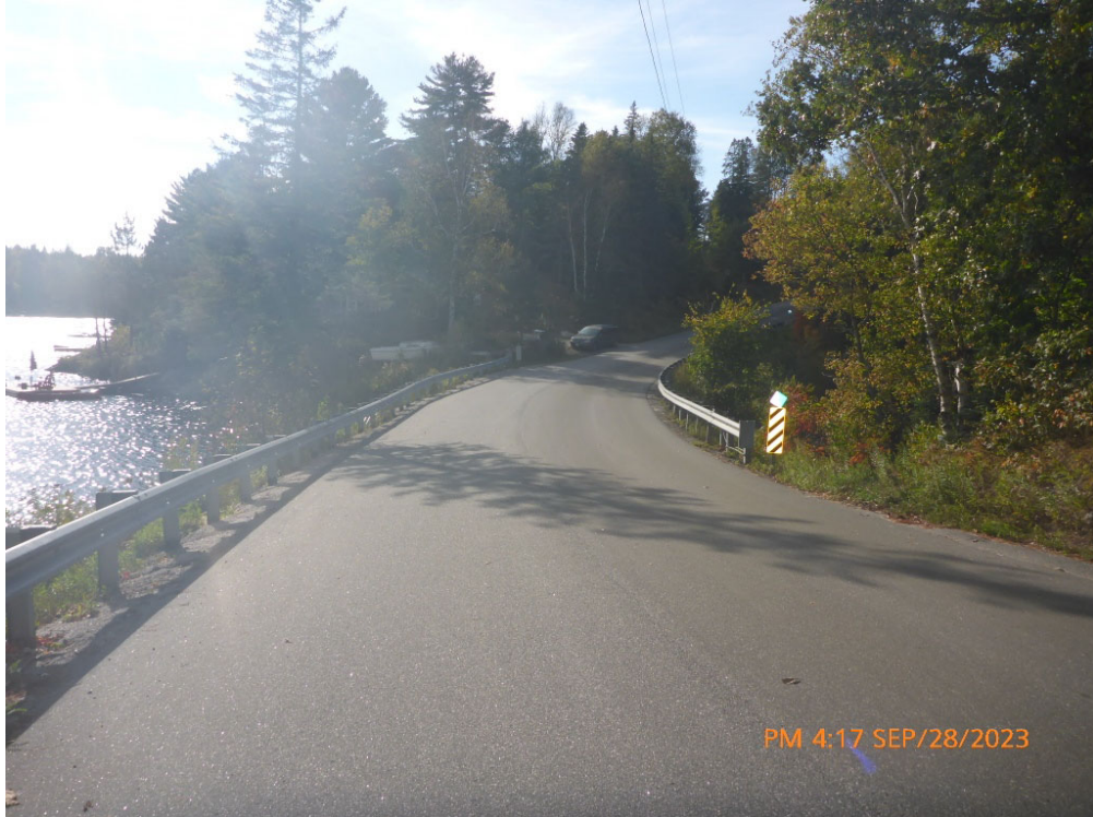
Comments: LOOKING WEST AT ROADWAY OVER CULVERT Path: P:\McKellar\2023\P1080309.jpg
