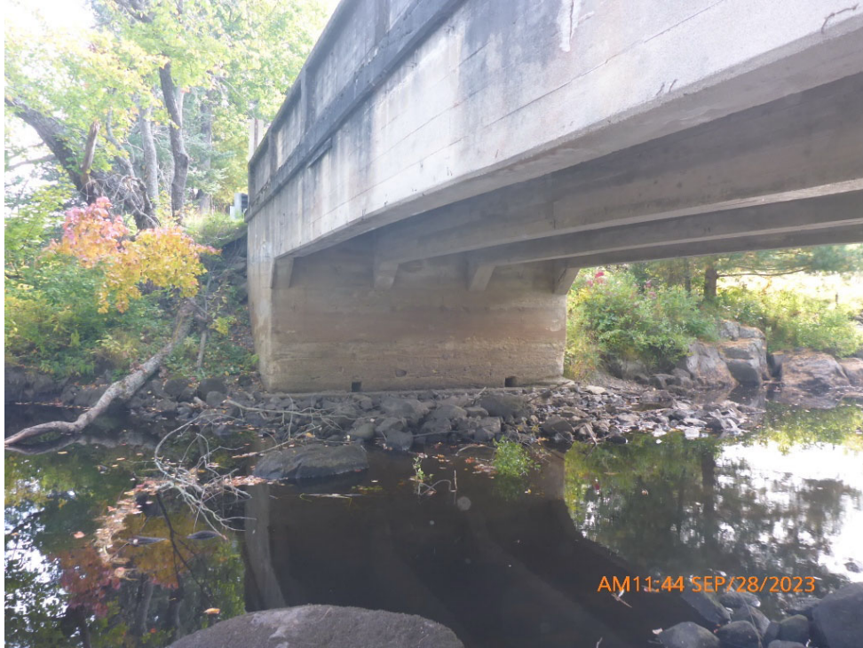
Comments: TYPICAL EAST ABUTMENT
