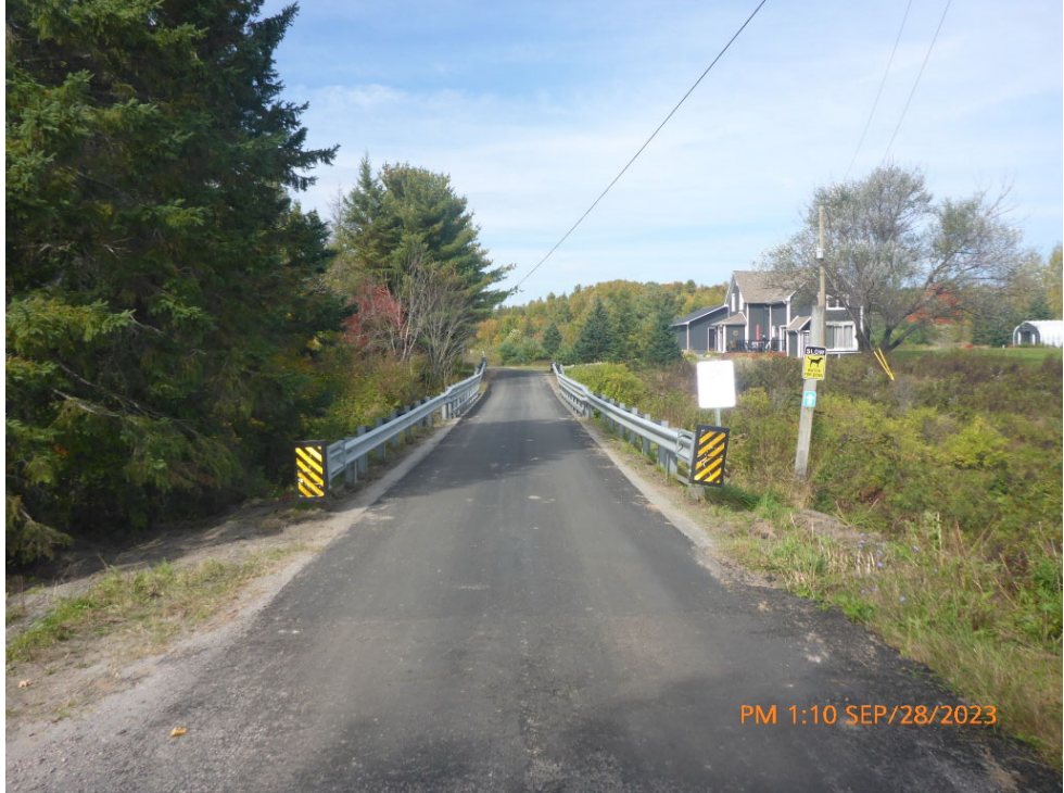
Comments: LOOKING NORTH AT BRIDGE Path: P:\McKellar\2023\P1080206.jpg
