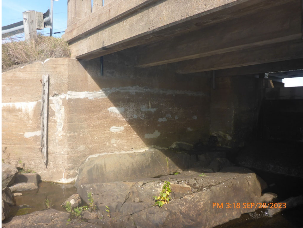
Comments: TYPICAL NORTH ABUTMENT Path: P:\McKellar\2023\P1080284.jpg
