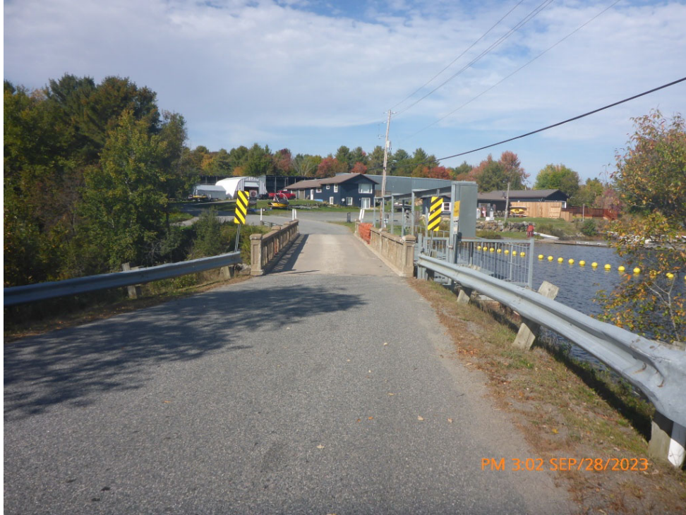
Comments: LOOKING NORTH AT BRIDGE Path: P:\McKellar\2023\P1080263.jpg
