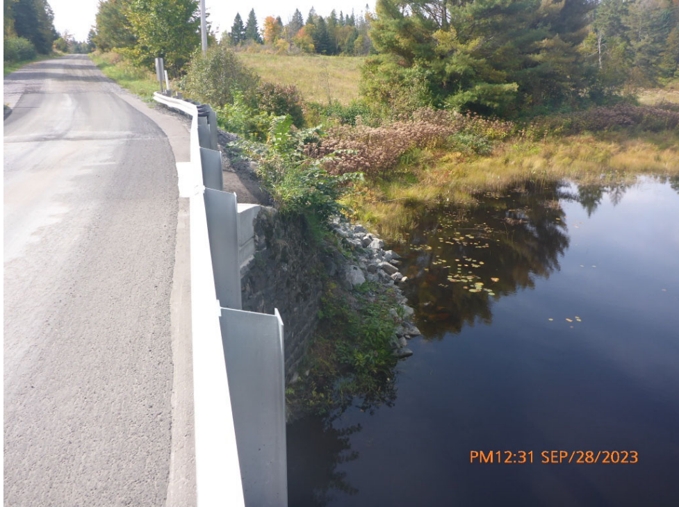
Comments: ROCK PROTECTION PROVIDED IN SOUTHWEST QUADRANT
