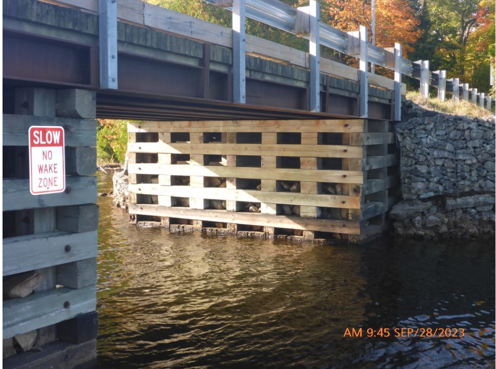
Comments: TYPICAL WEST ABUTMENT
