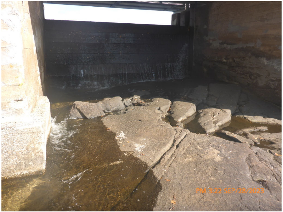
Comments: WATERCOURSE UNDER BRIDGE
