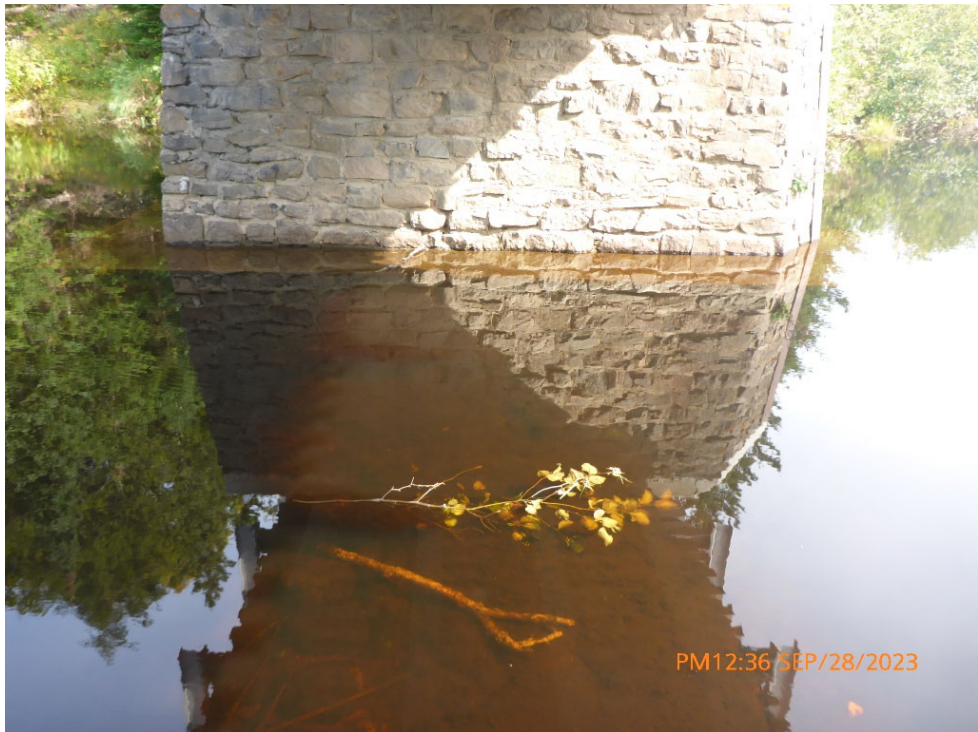
Comments: WATERCOURSE UNDER BRIDGE
