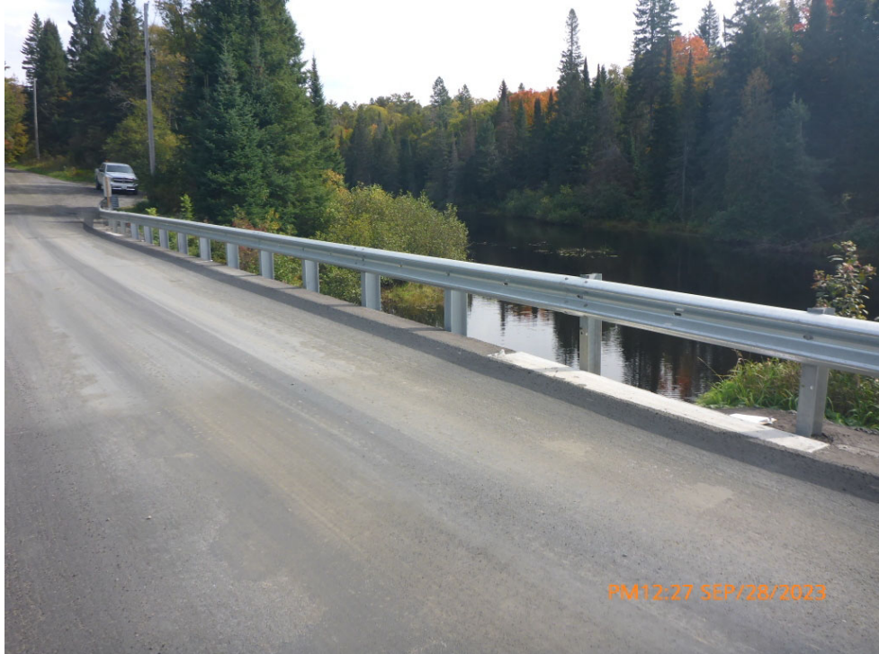
Comments: NEW GUIDE RAIL INSTALLED OVER DECK
