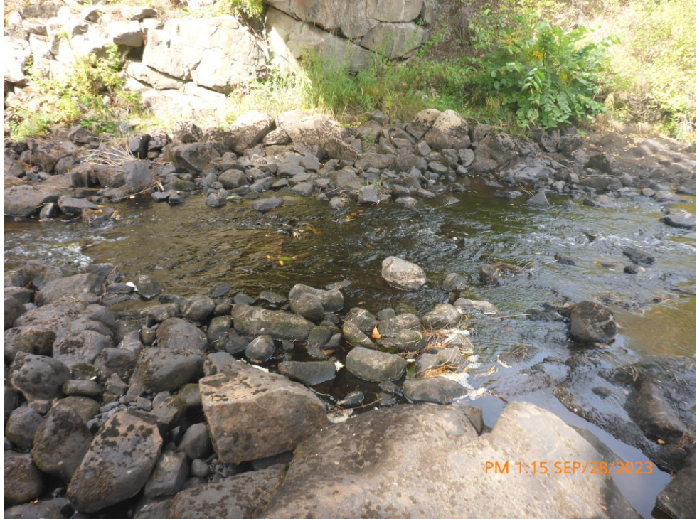
Comments: WATERCOURSE UNDER BRIDGE Path: P:\McKellar\2023\P1080218.jpg
