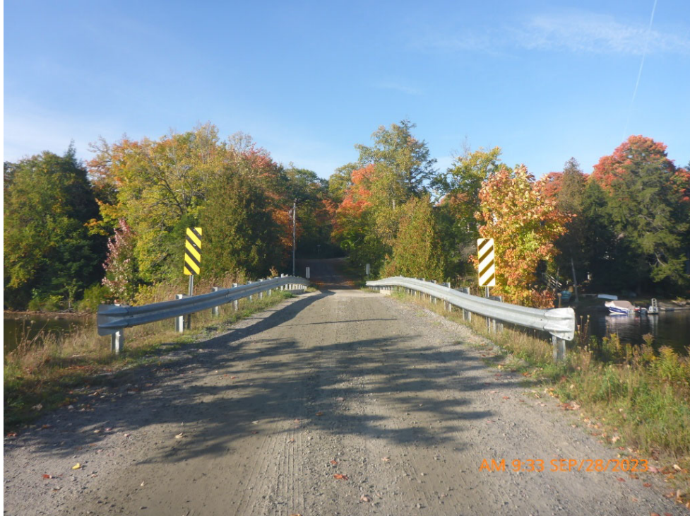
Comments: LOOKING WEST AT BRIDGE
