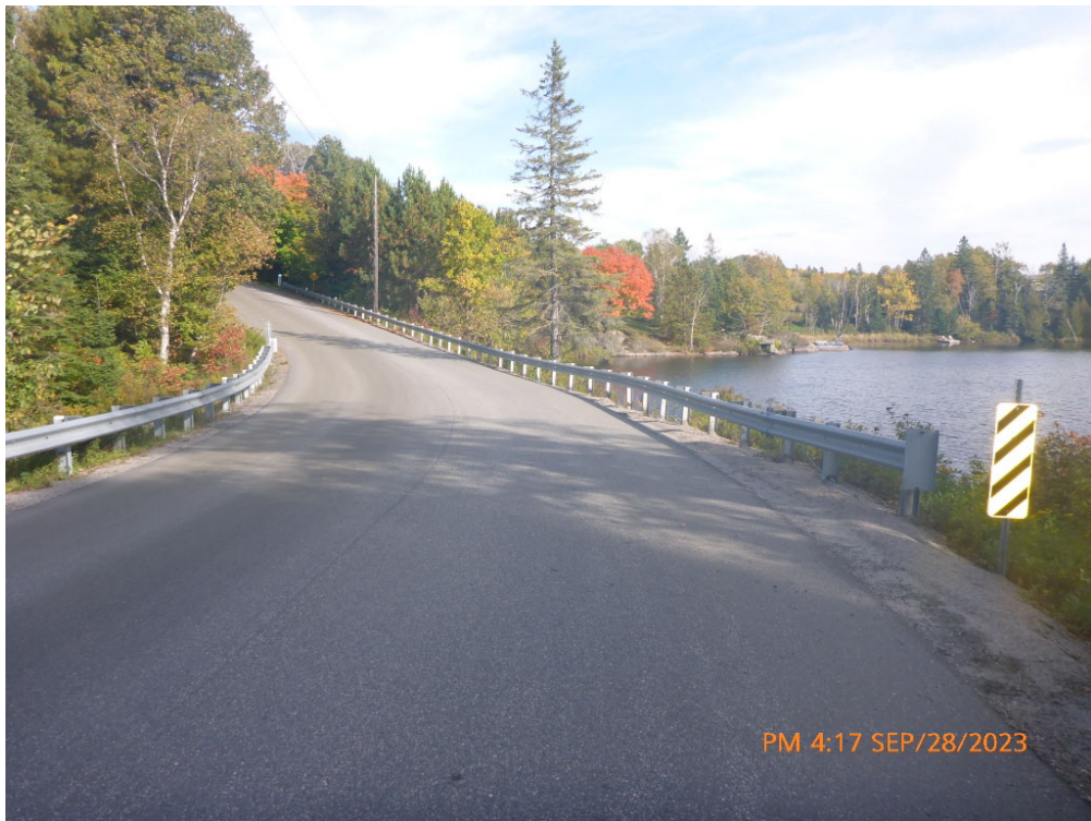
Comments: LOOKING EAST AT ROADWAY OVER CULVERT Path: P:\McKellar\2023\P1080310.jpg
