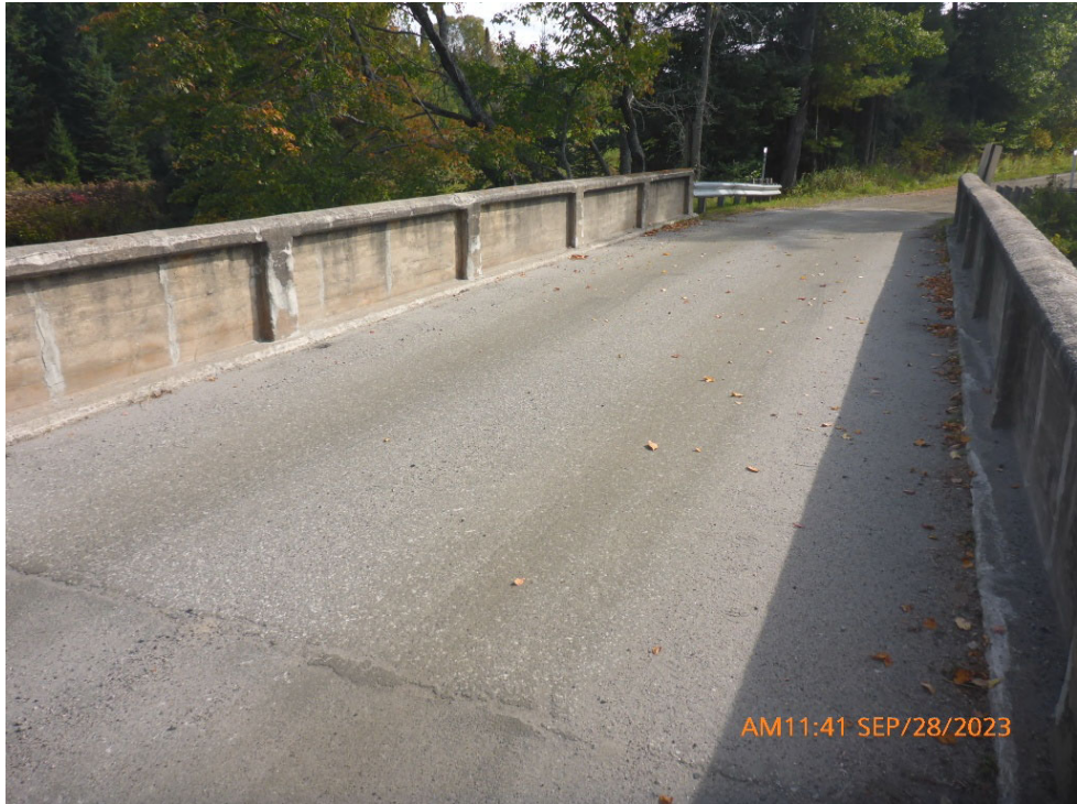
Comments: TYPICAL DECK WEARING SURFACE
