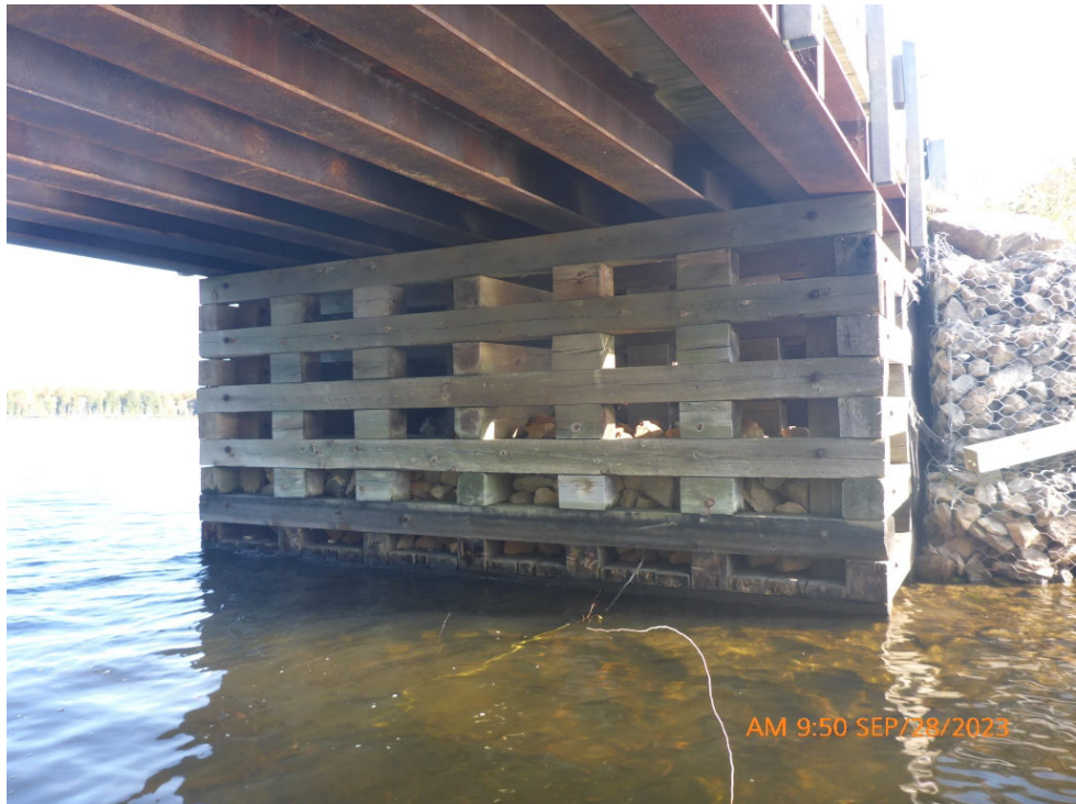
Comments: TYPICAL EAST ABUTMENT
