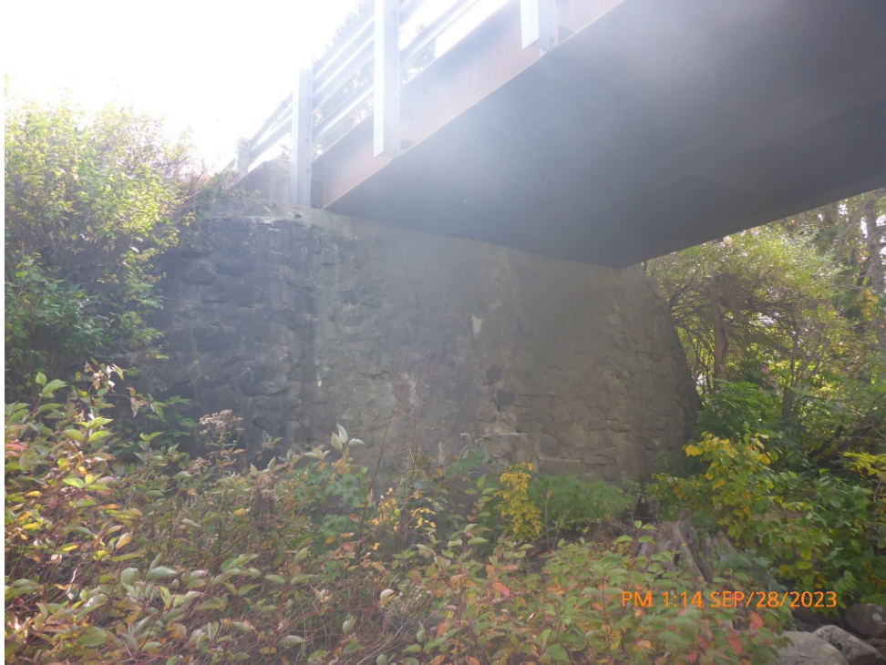
Comments: TYPICAL SOUTH ABUTMENT Path: P:\McKellar\2023\P1080216.jpg
