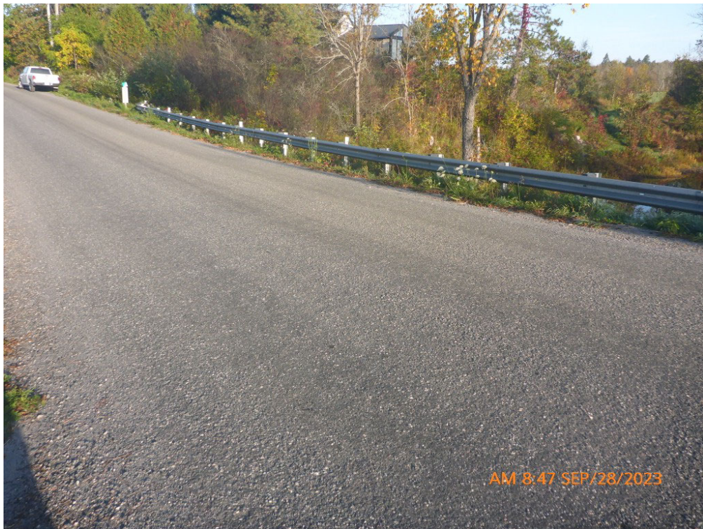
Comments: TYPICAL WEARING SURFACE Path: P:\McKellar\2023\P1080083.jpg
