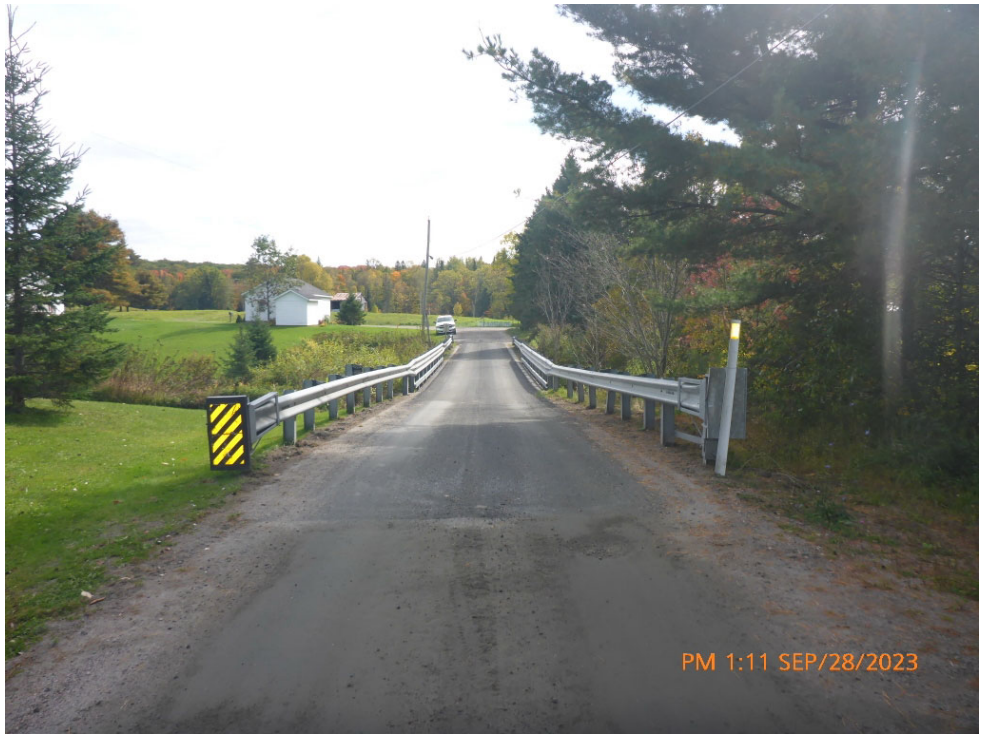
Comments: LOOKING SOUTH AT BRIDGE Path: P:\McKellar\2023\P1080207.jpg
