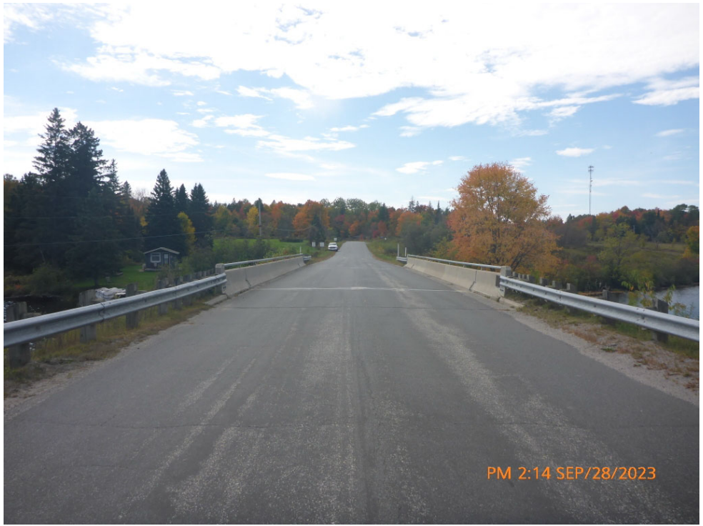
Comments: LOOKING SOUTH AT BRIDGE Path: P:\McKellar\2023\P1080235.jpg
