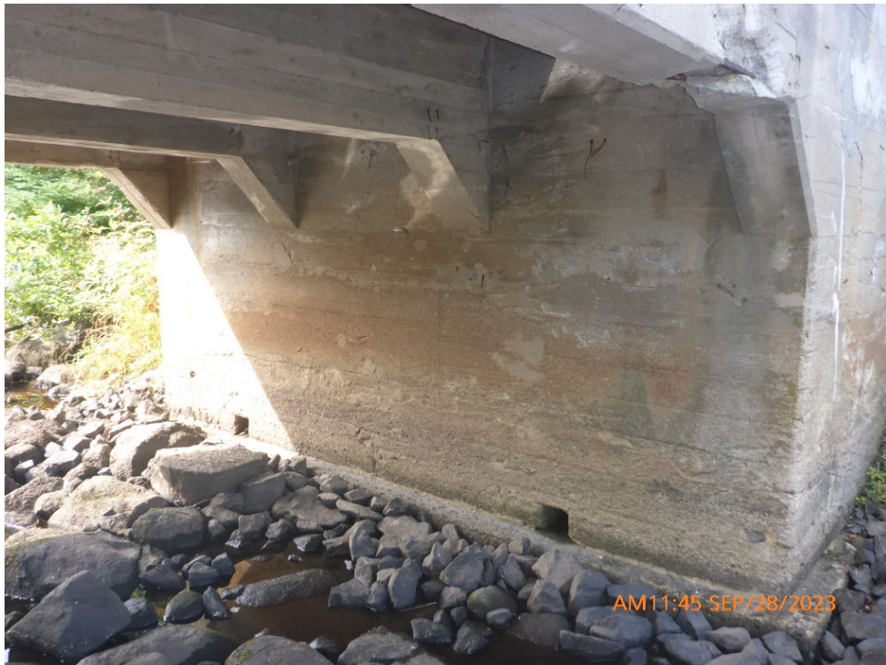
Comments: TYPICAL WEST ABUTMENT
