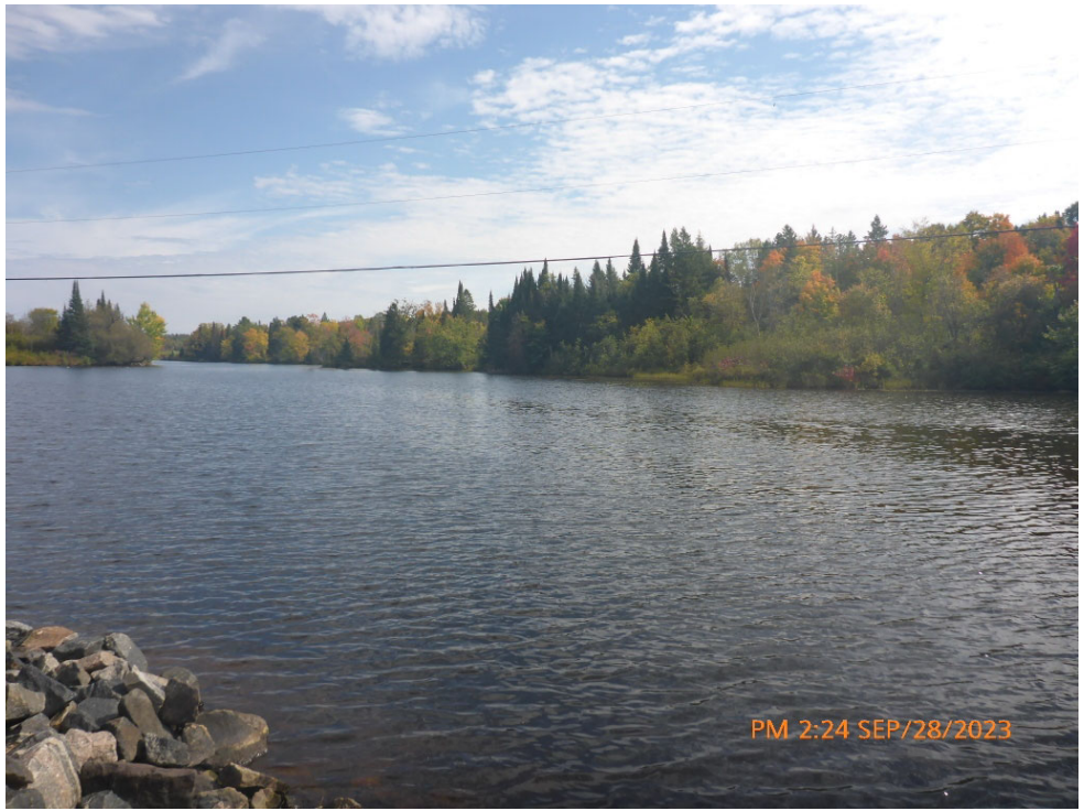
Comments: LOOKING EAST UPSTREAM Path: P:\McKellar\2023\P1080253.jpg
