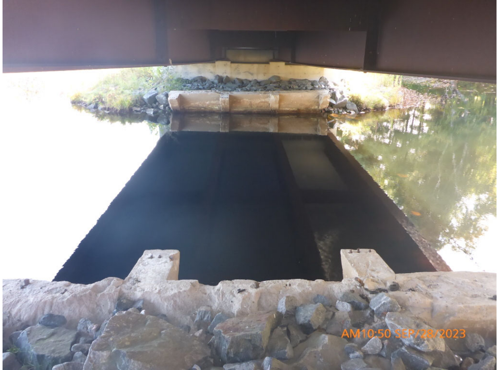
Comments: WATERCOURSE UNDER BRIDGE Path: P:\McKellar\2023\P1080141.jpg
