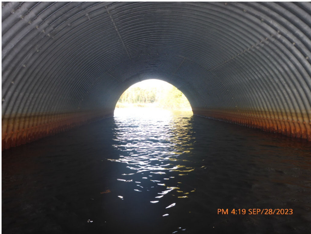
Comments: LOOKING NORTH THROUGH BARREL
