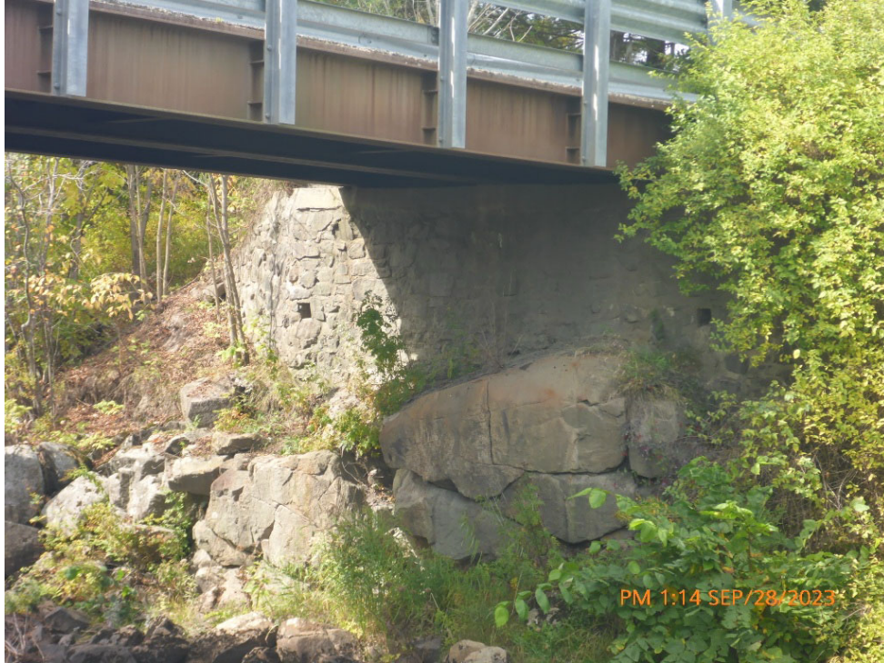
Comments: TYPICAL NORTH ABUTMENT Path: P:\McKellar\2023\P1080215.jpg
