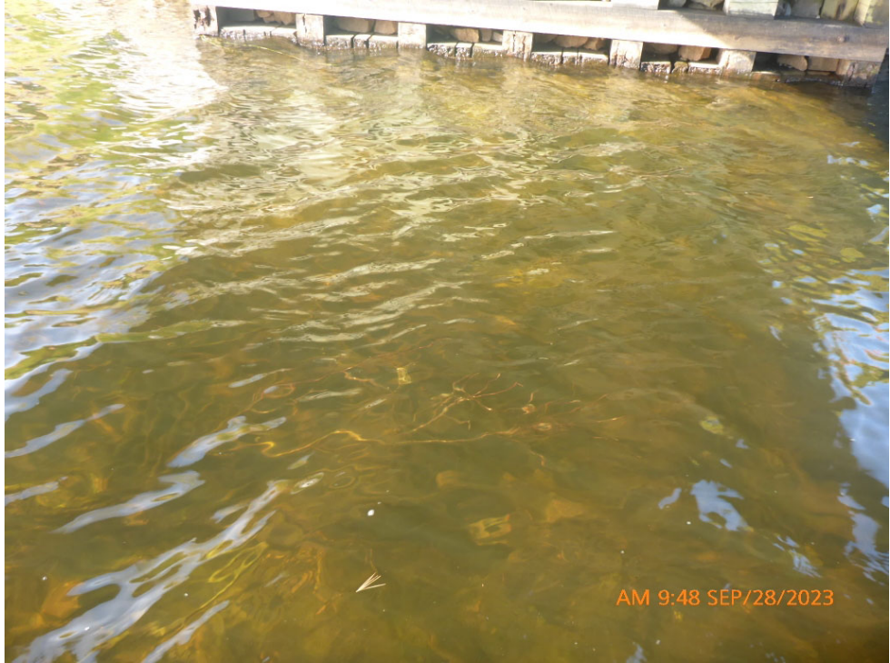
Comments: WATERCOURSE UNDER BRIDGE Path: P:\McKellar\2023\P1080114.jpg
