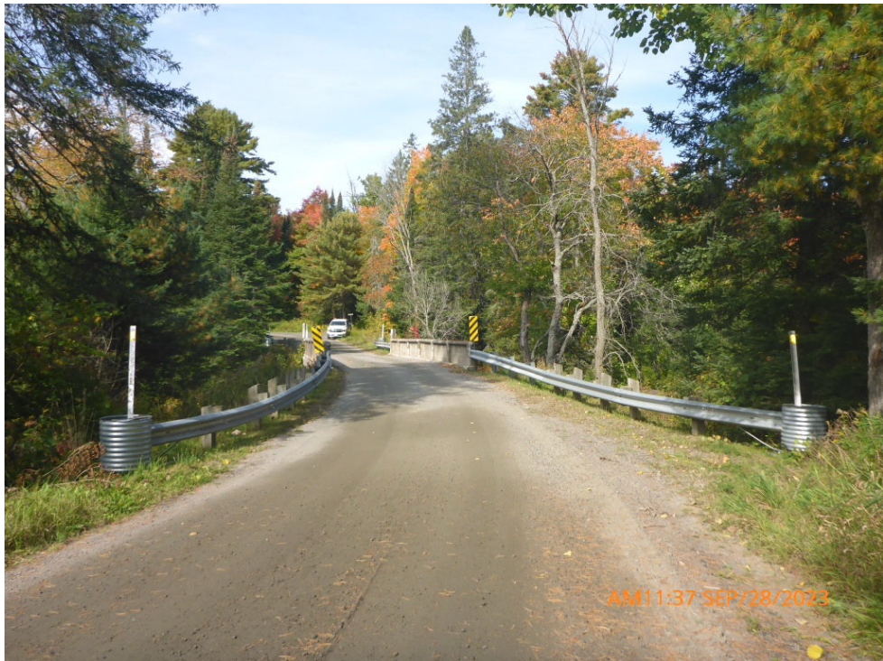
Comments: LOOKING WEST AT BRIDGE
