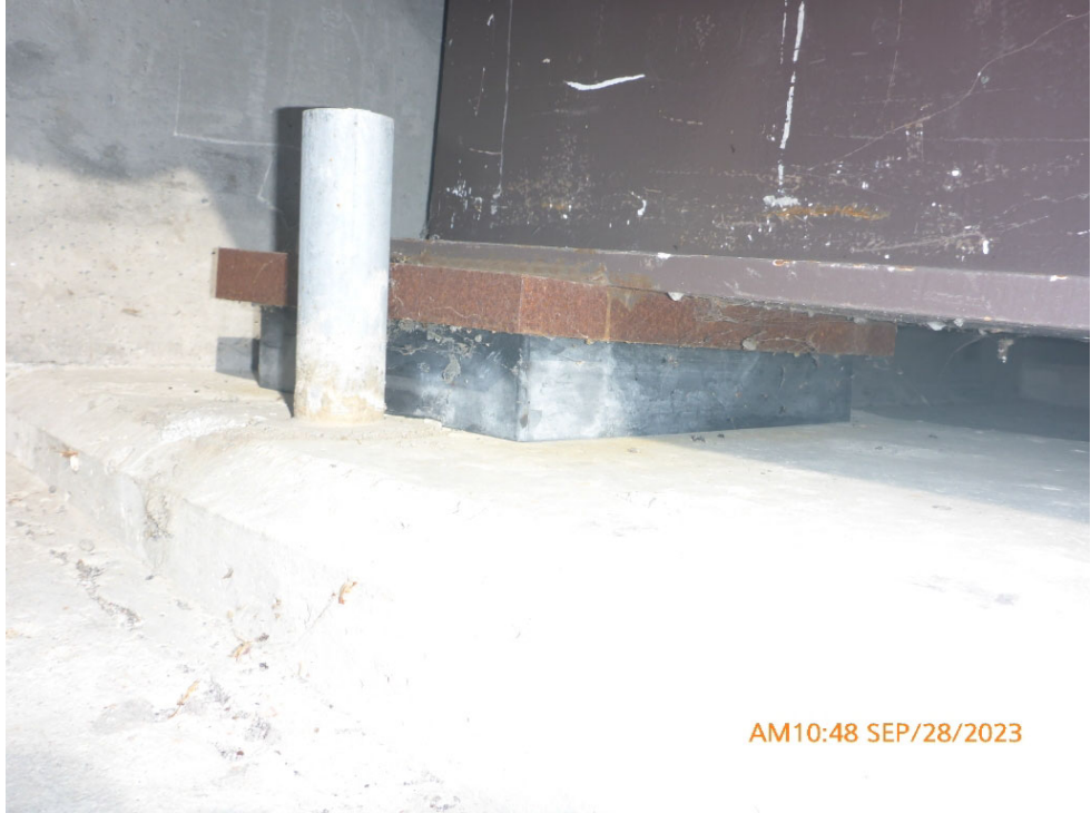
Comments: TYPICAL ABUTMENT BEARING Path: P:\McKellar\2023\P1080137.jpg
