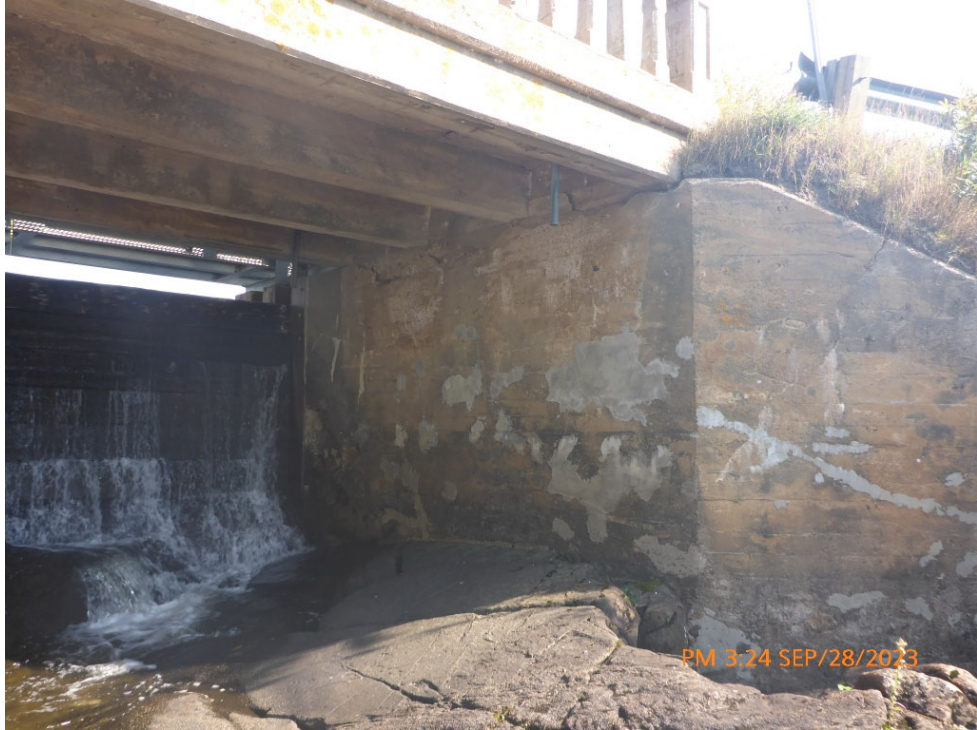
Comments: TYPICAL SOUTH ABUTMENT
