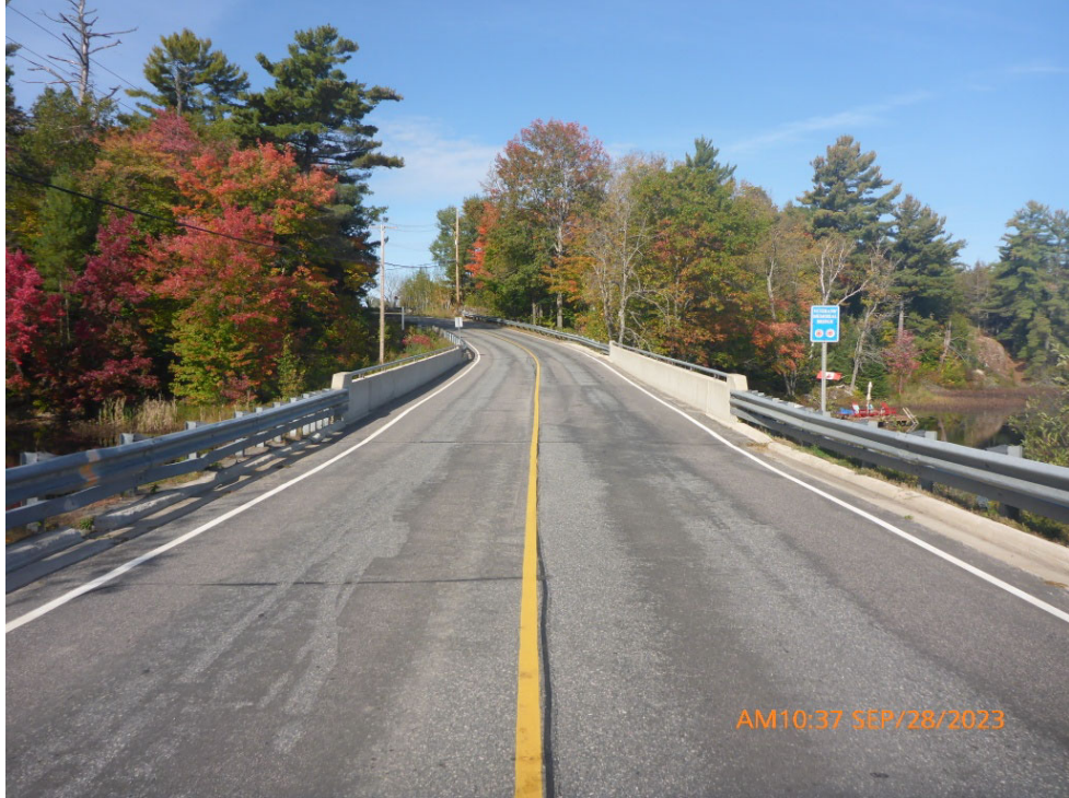
Comments: LOOKING WEST AT BRIDGE
