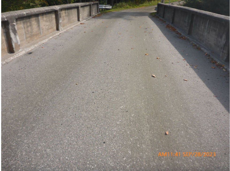
Comments: LIGHT FLUSHING OF DECK WEARING SURFACE
