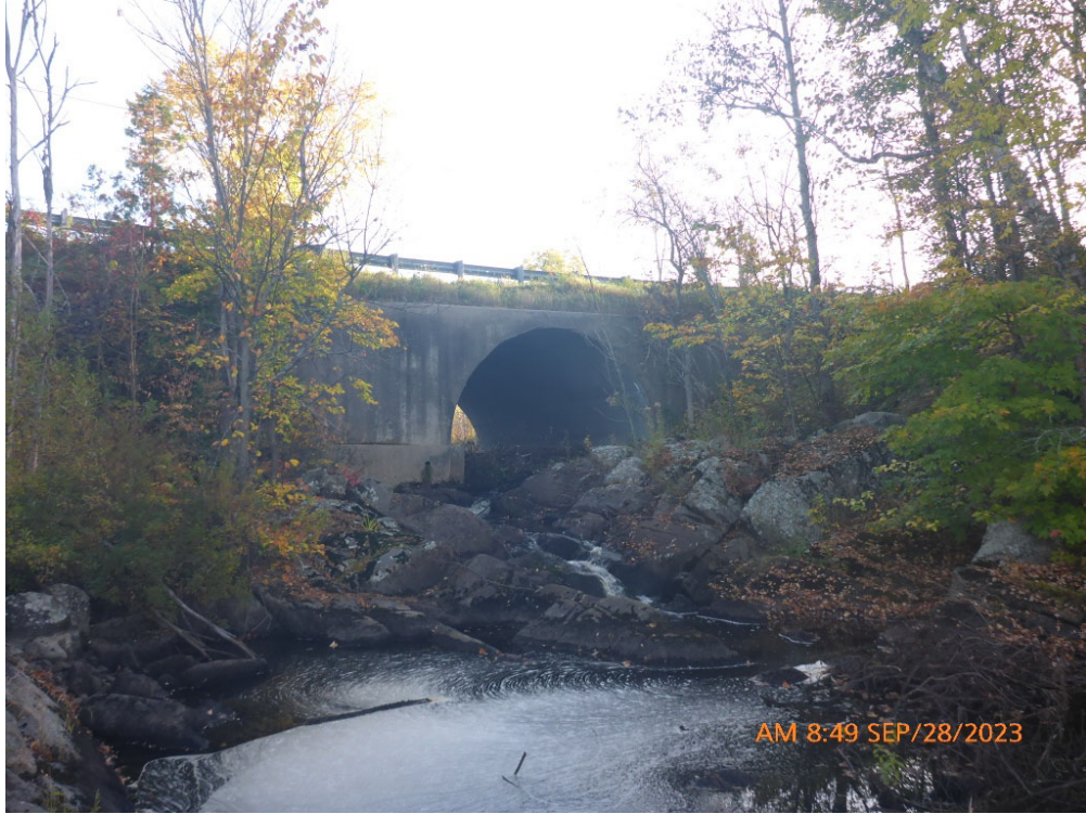
Comments: SOUTH ELEVATION Path: P:\McKellar\2023\P1080086.jpg
