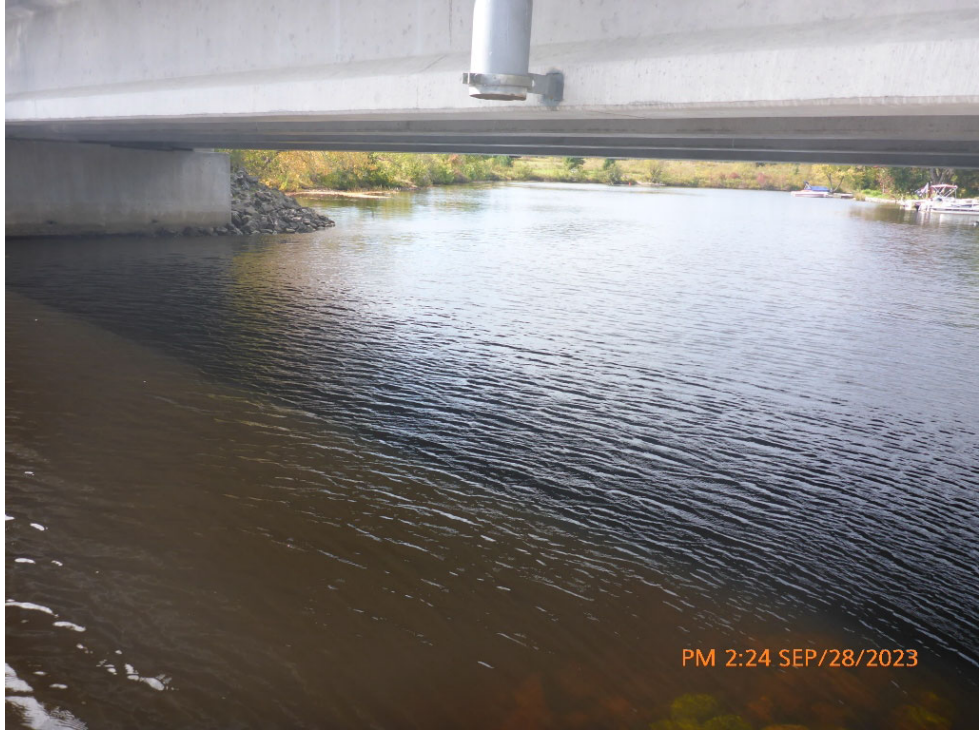
Comments: WATERCOURSE UNDER BRIDGE Path: P:\McKellar\2023\P1080252.jpg
