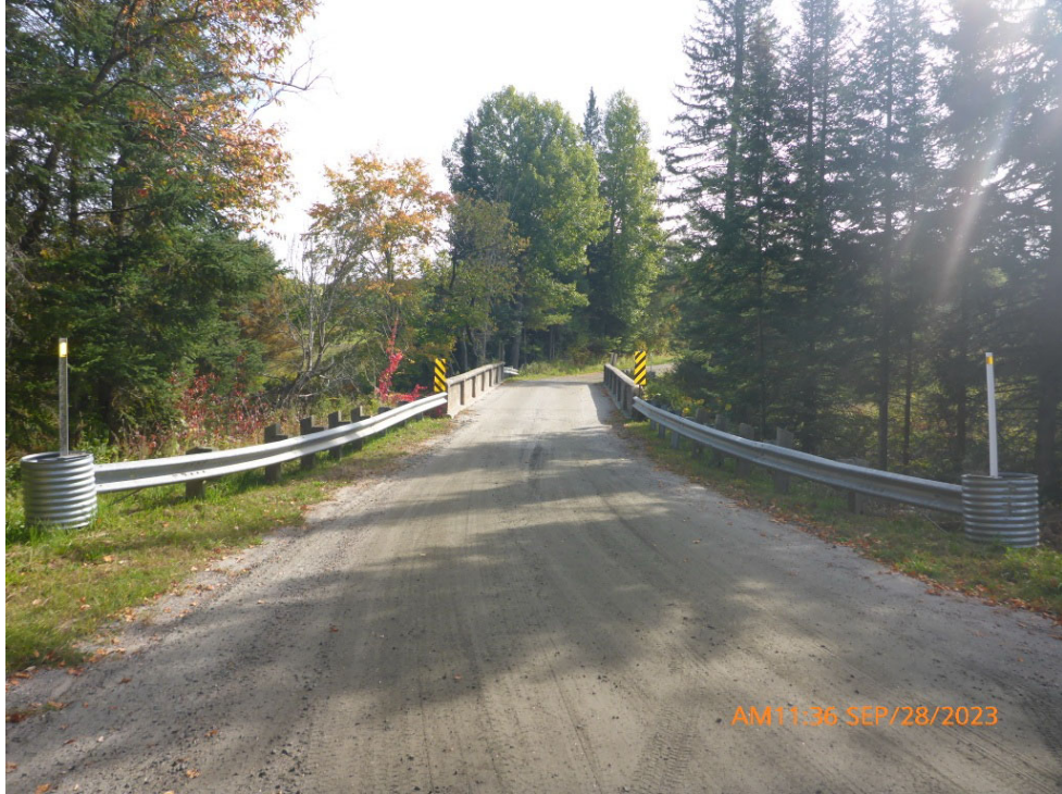
Comments: LOOKING EAST AT BRIDGE
