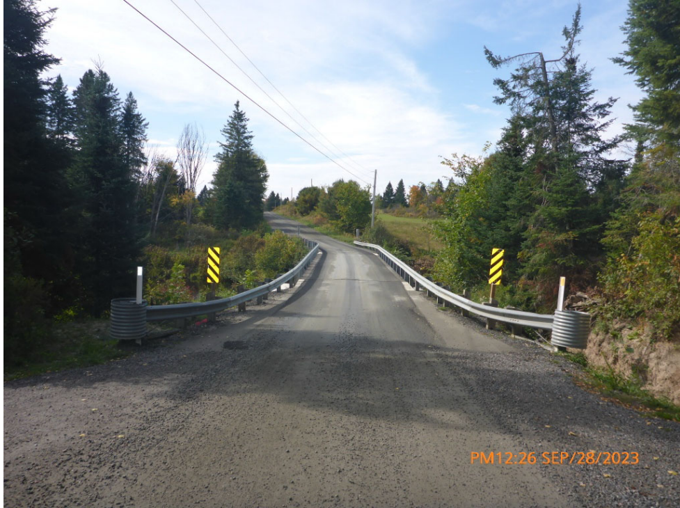
Comments: LOOKING SOUTH AT BRIDGE
