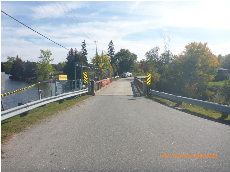
Comments: LOOKING SOUTH AT BRIDGE Path: P:\McKellar\2023\P1080264.jpg
