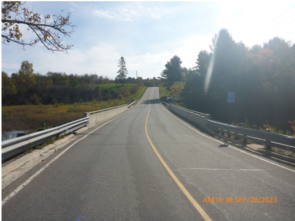
Comments: LOOKING EAST AT BRIDGE
