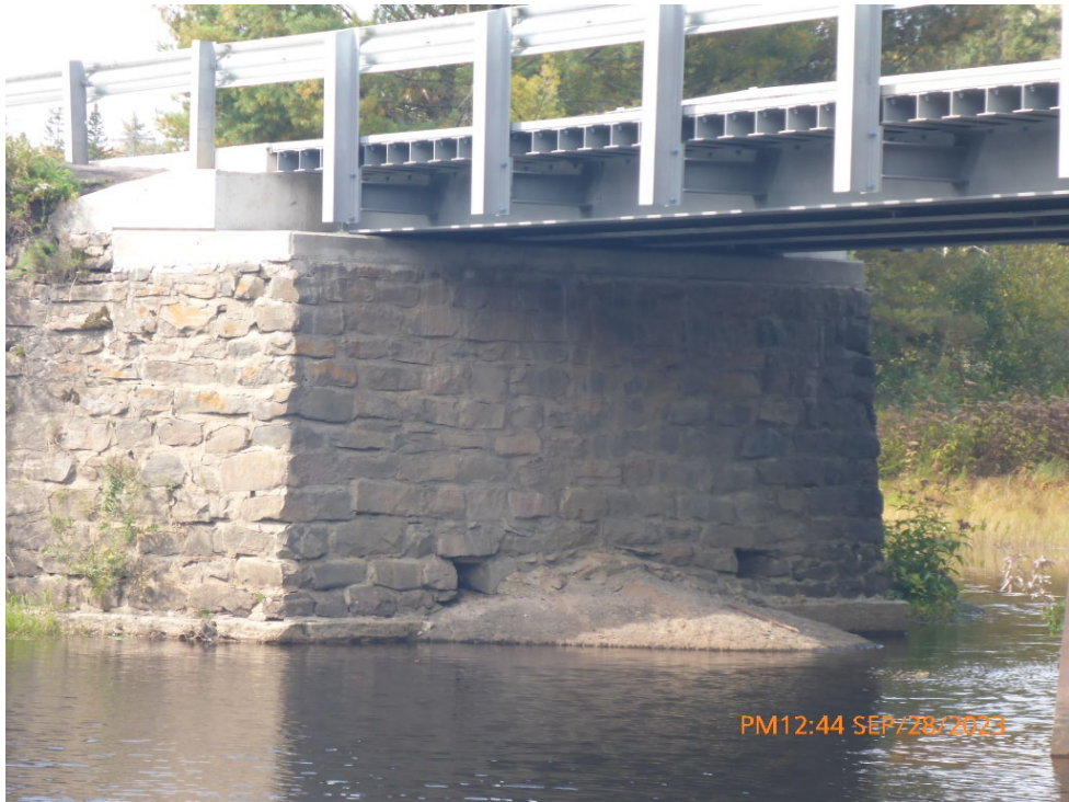
Comments: TYPICAL SOUTH ABUTMENT
