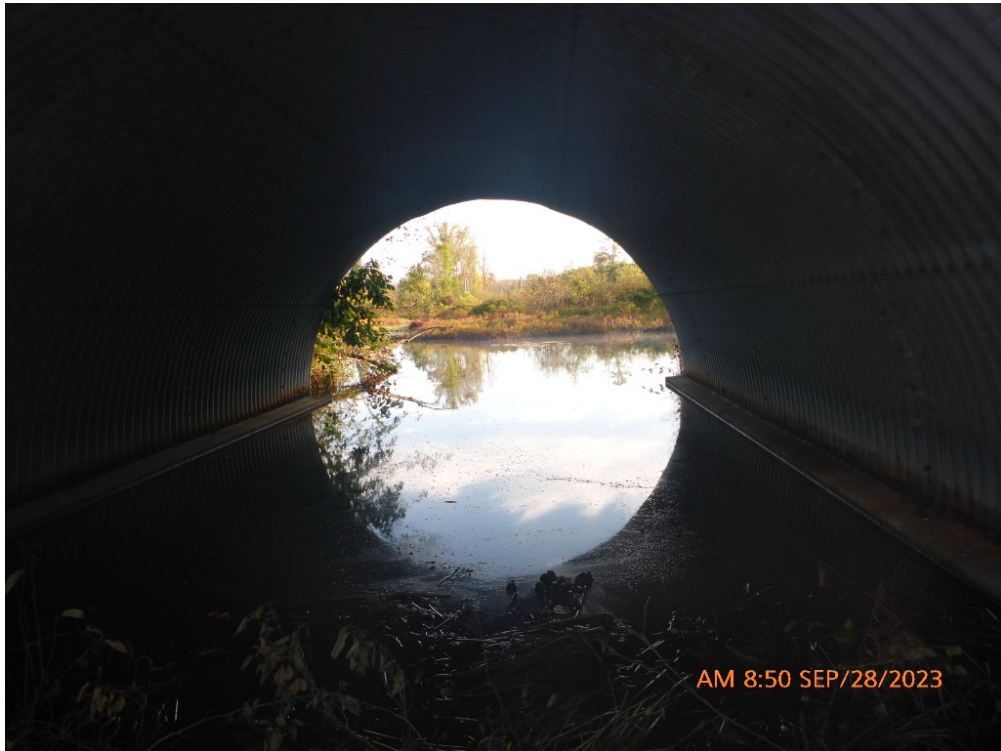
Comments: LOOKING NORTH THROUGH BARREL
