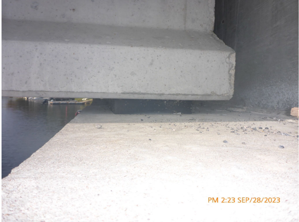
Comments: TYPICAL ABUTMENT BEARING
