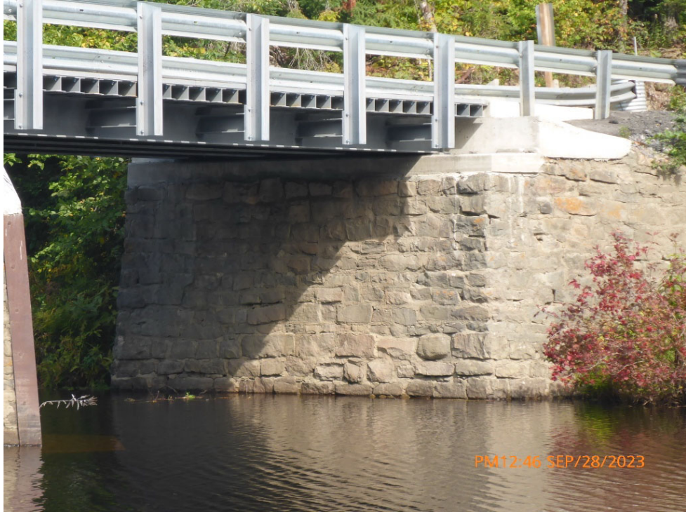
Comments: TYPICAL NORTH ABUTMENT Path: P:\McKellar\2023\P1080201.jpg
