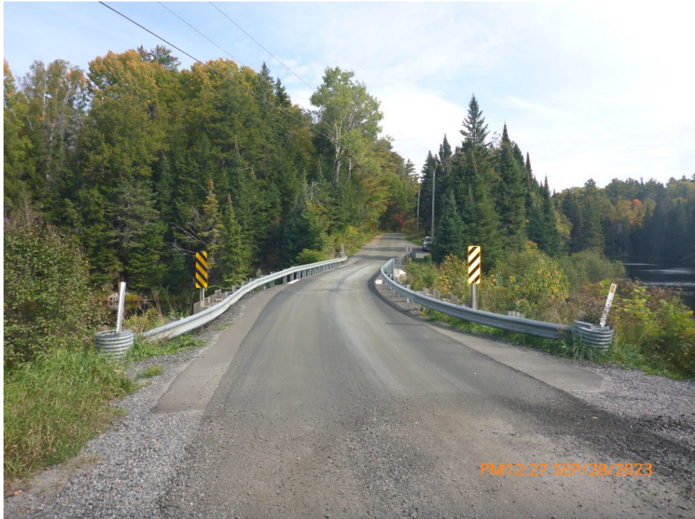
Comments: LOOKING NORTH AT BRIDGE
