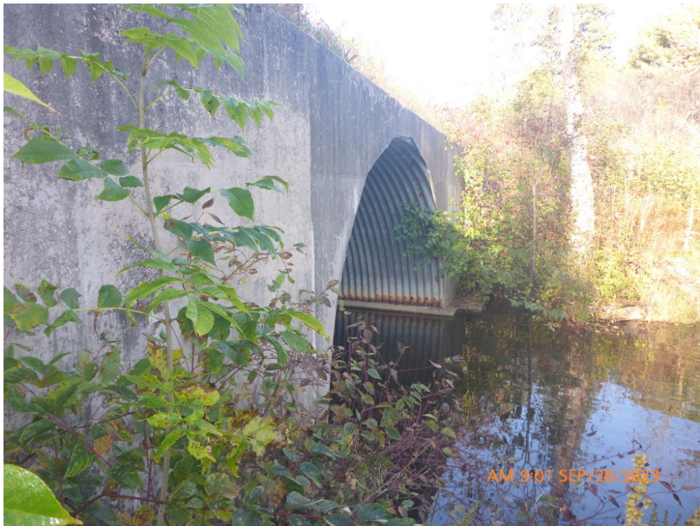
Comments: NORTH ELEVATION Path: P:\McKellar\2023\P1080094.jpg
