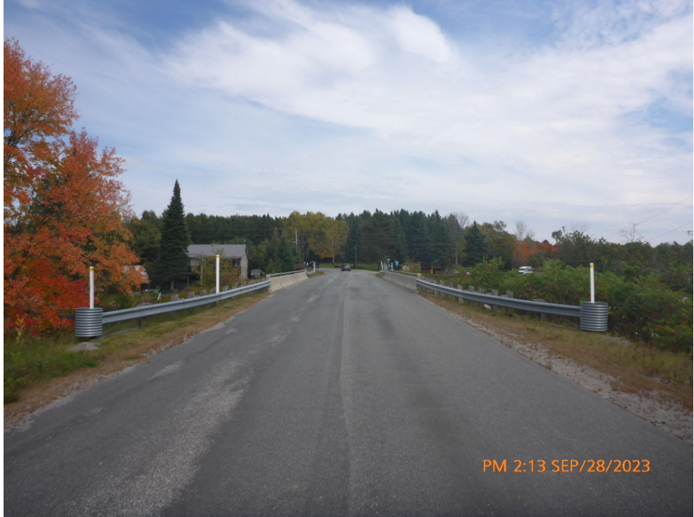
Comments: LOOKING NORTH AT BRIDGE Path: P:\McKellar\2023\P1080234.jpg
