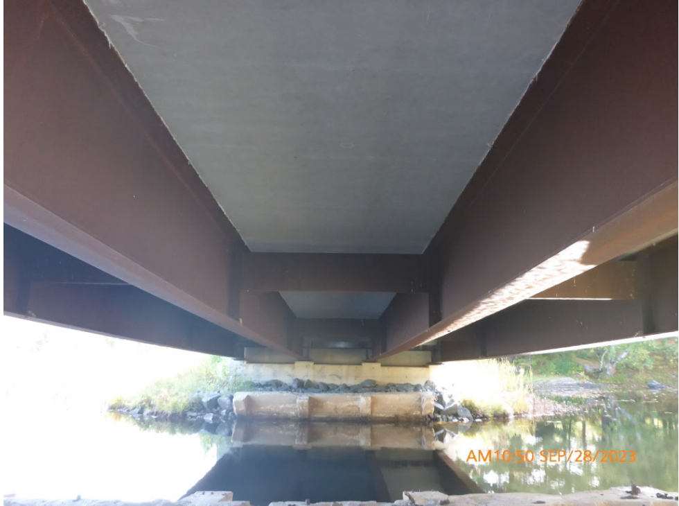
Comments: TYPICAL SOFFIT Path: P:\McKellar\2023\P1080140.jpg
