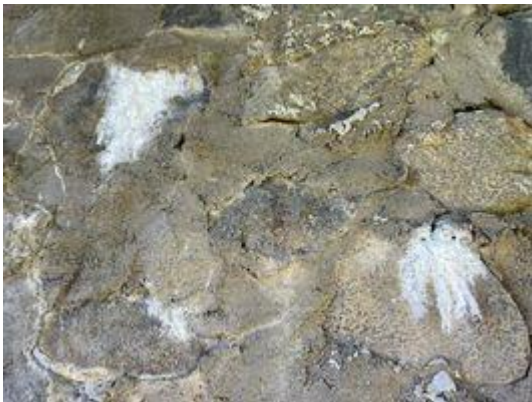
Photo 3: Efflorescence
